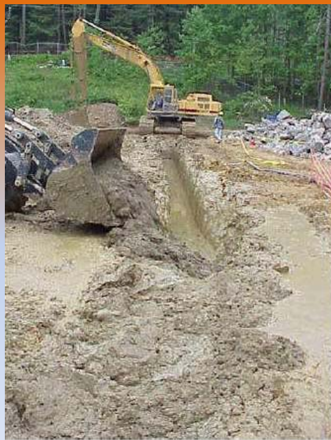
SCB Backfill being placed in the Trench
