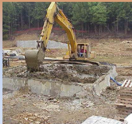
Mixing SCB Backfill in an Enclosed mixing Area
