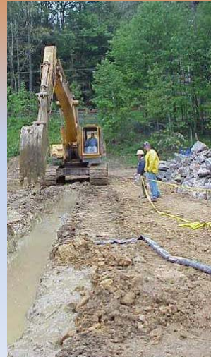
Trenching Under Bentonite Slurry
