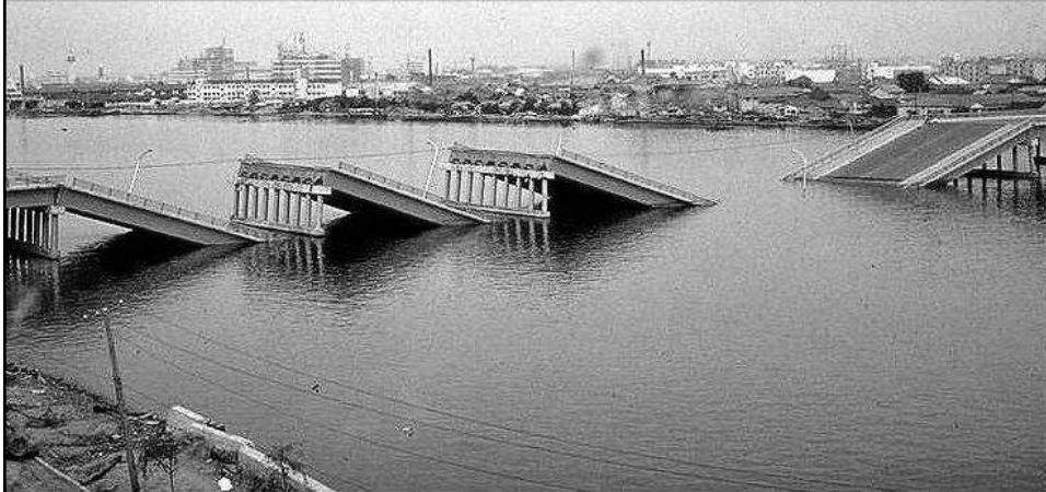
Showa River bridge following 1964 Niigata earthquake
